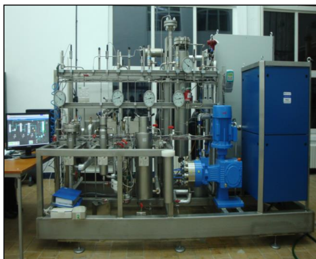
Figure 1. Experimental plant for supercritical fluid extraction of walnut green husk
